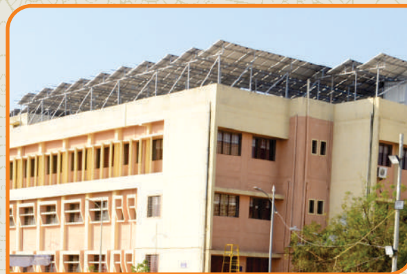
Solar Panel Installation
